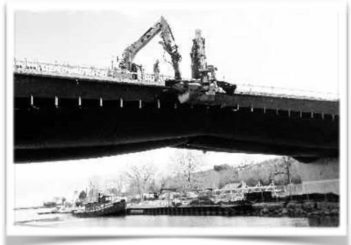
The current bridge being taken down, February 2017
