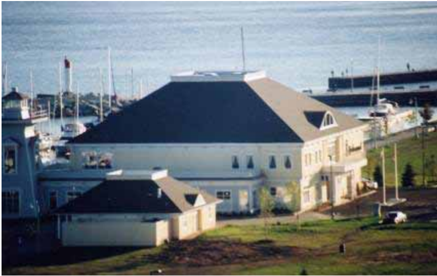
Bronte Outer Harbour – Lighthouse Restaurant finished 2003
