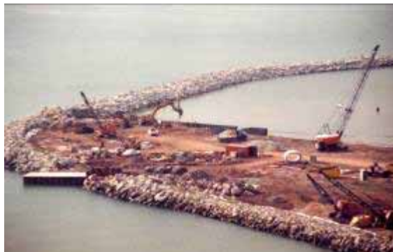
Bronte Outer Harbour – preparing Marina 2001
