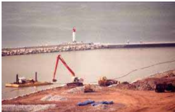
Bronte Outer Harbour – laying stone 2001
