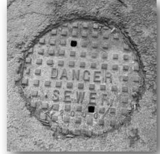
J W 159 DANGER SEWER 2000
