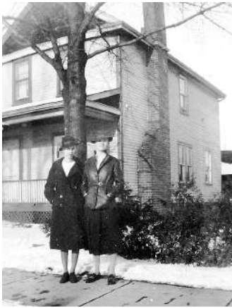
371 Kerr St. 1935 before present Insulbrick cladding
