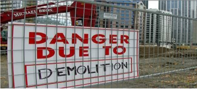
Condo development on site of demolished Addison-on-Bay art deco building
