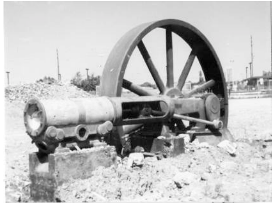
Wheel before the move across Cornwall Road.
