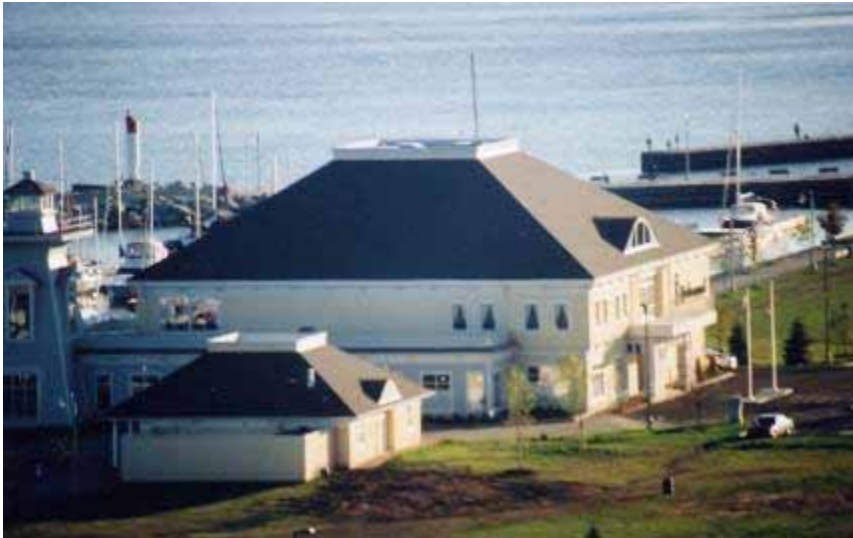
Bronte Outer Harbour – Lighthouse Restaurant finished 2003
