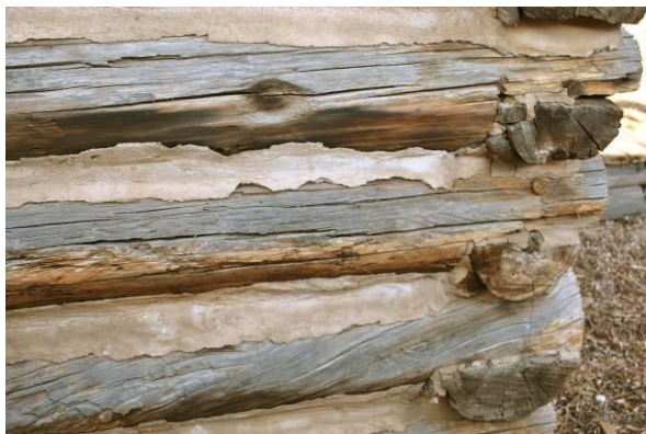
Chinking between logs and, corners
