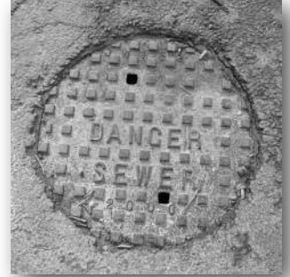
J W 159 DANGER SEWER 2000
