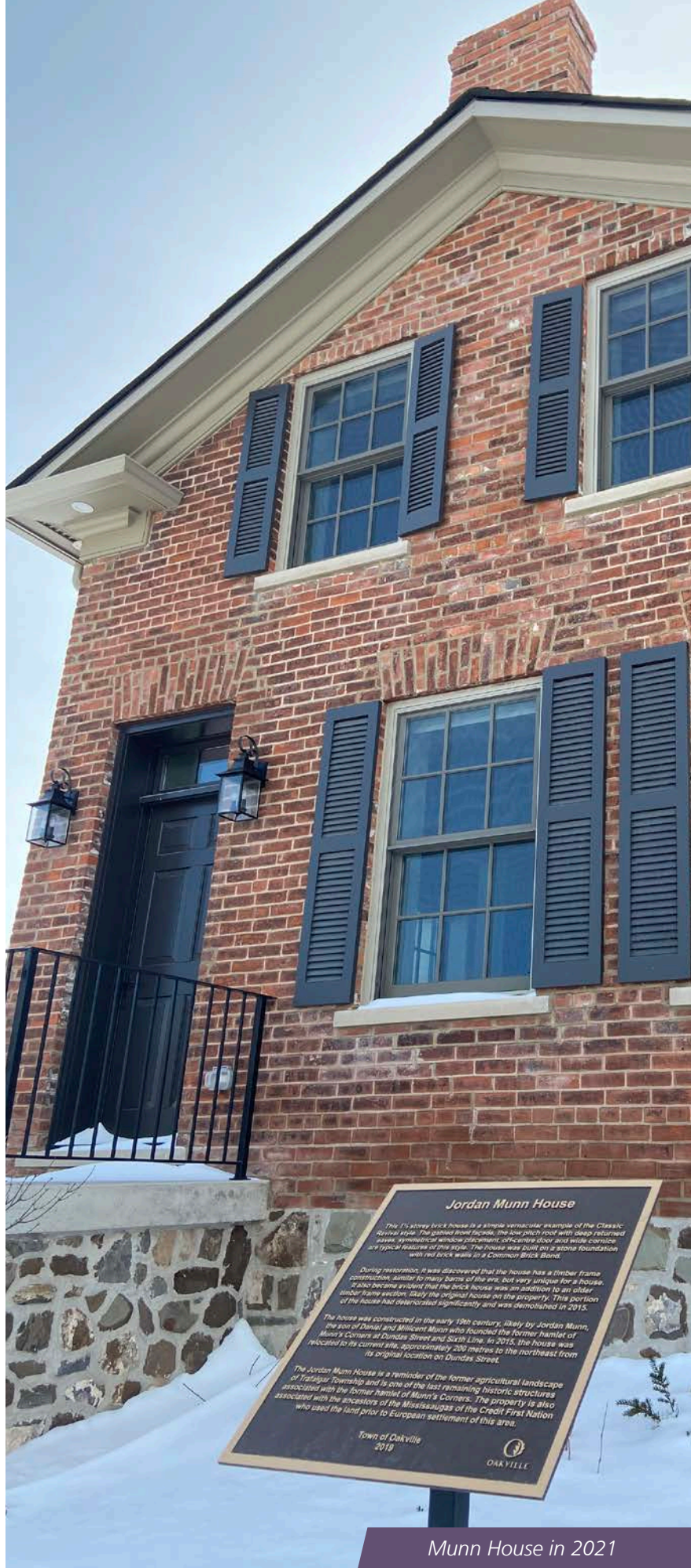
Original timber frame structure exposed during restoration
