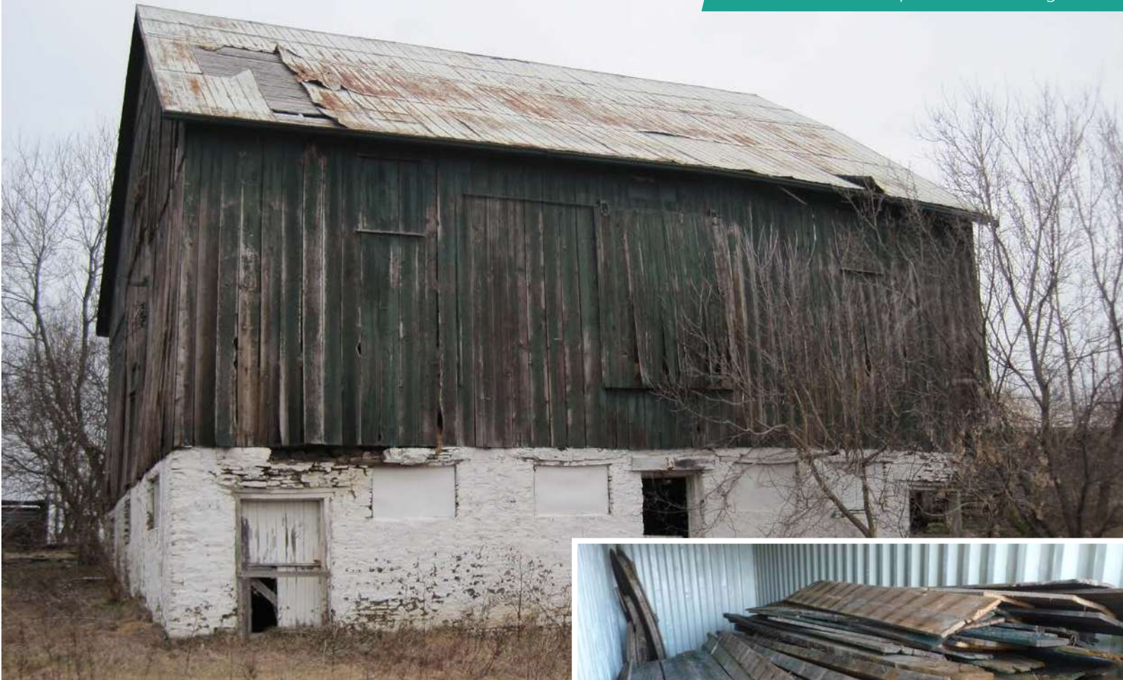
Featherstone Barn prior to dismantling
